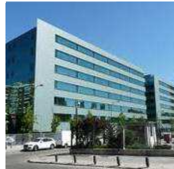
Office Building Branch offices
